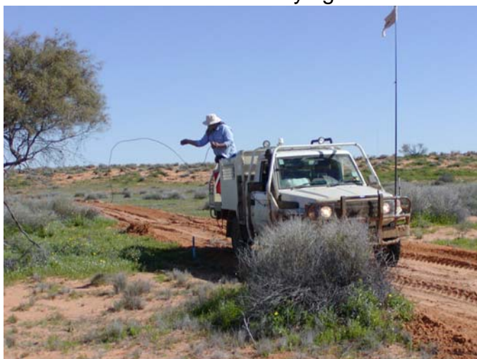
Plate 1 Light 4WD laying cables.
